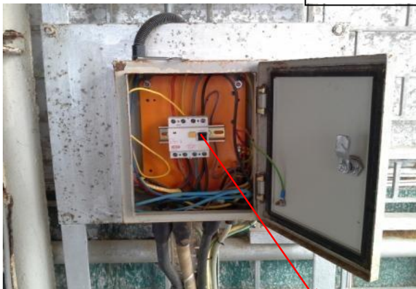
Pic.9 Main power Switch
